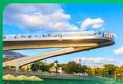
Floating Bridge Moscow
