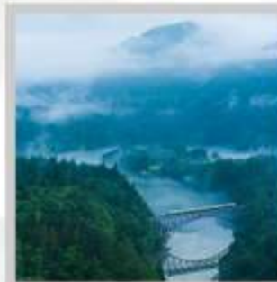
"TADAMI FIRST BRIDGE"
